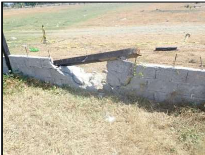
Figure 2. The aircraft collided with the airport perimeter fence.
