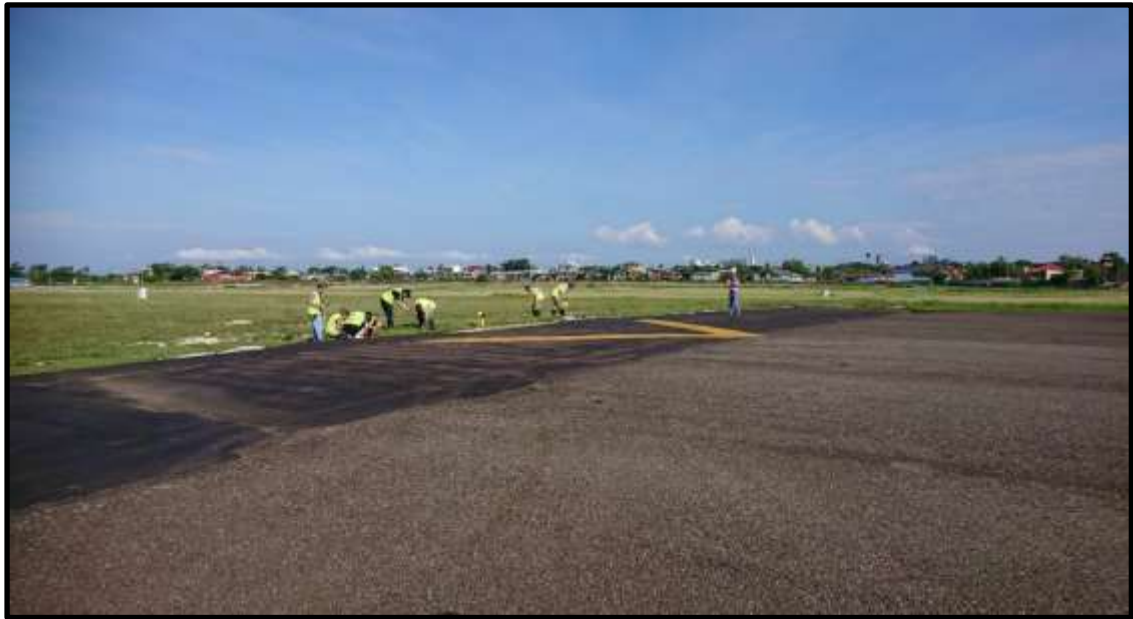
Figure 10 - The edge of the paved portion before the threshold of RWY 22.
