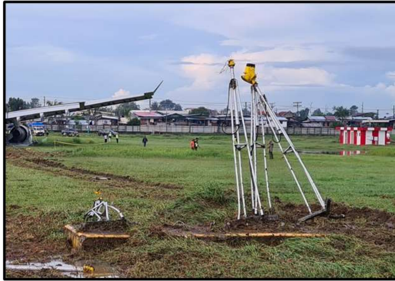
Figure 2 - RPVM RWY 04 Approach lights.
