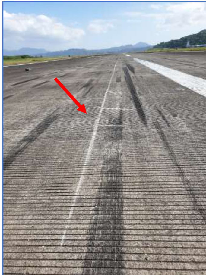
Figure 1: Shows the propeller strike and runway scrape marks.
